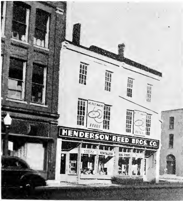
The Hanna Building at the northwest corner of Barr and Columbia streets as it appeared in 1952 after the east one-third of the building was removed --Photo by Peter Certia.
